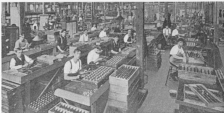
Fig. 34.—Assembling Receivers.
